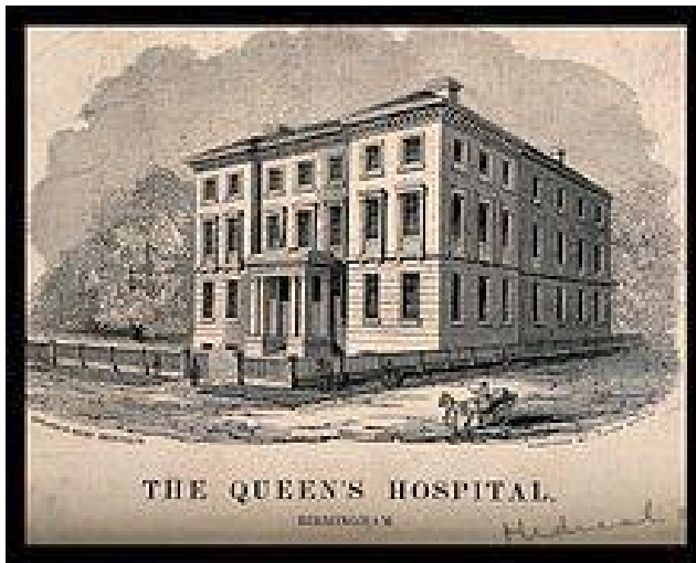
Fig. 4.6 The Queen's Hospital, Birmingham 1840
