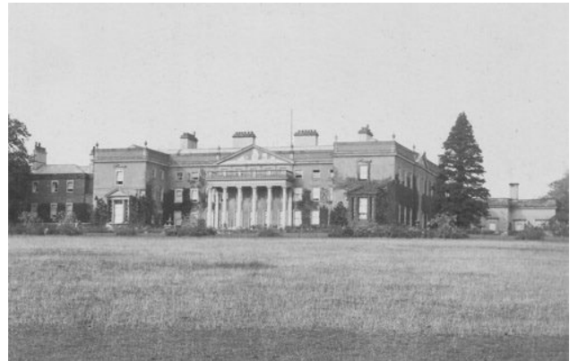
Fig. 2.3 Gopsall Hall South aspect
